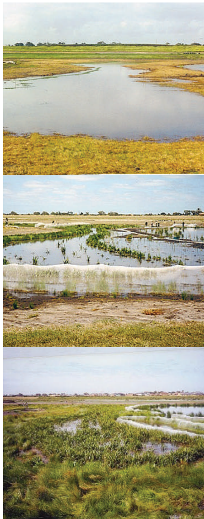
Photograph 4 This sequence of photographs, taken over a nine-month period at The Waterways, shows vegetation establishment in a constructed wetland from newly constructed and bare of native species on the top to well vegetated with a high cover of indigenous plants and minimal weeds on the bottom
